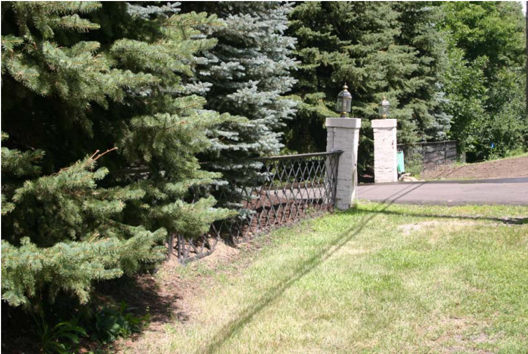
405 Bushaway Road – Decorative fence demarcating property boundary at Bushaway Road
