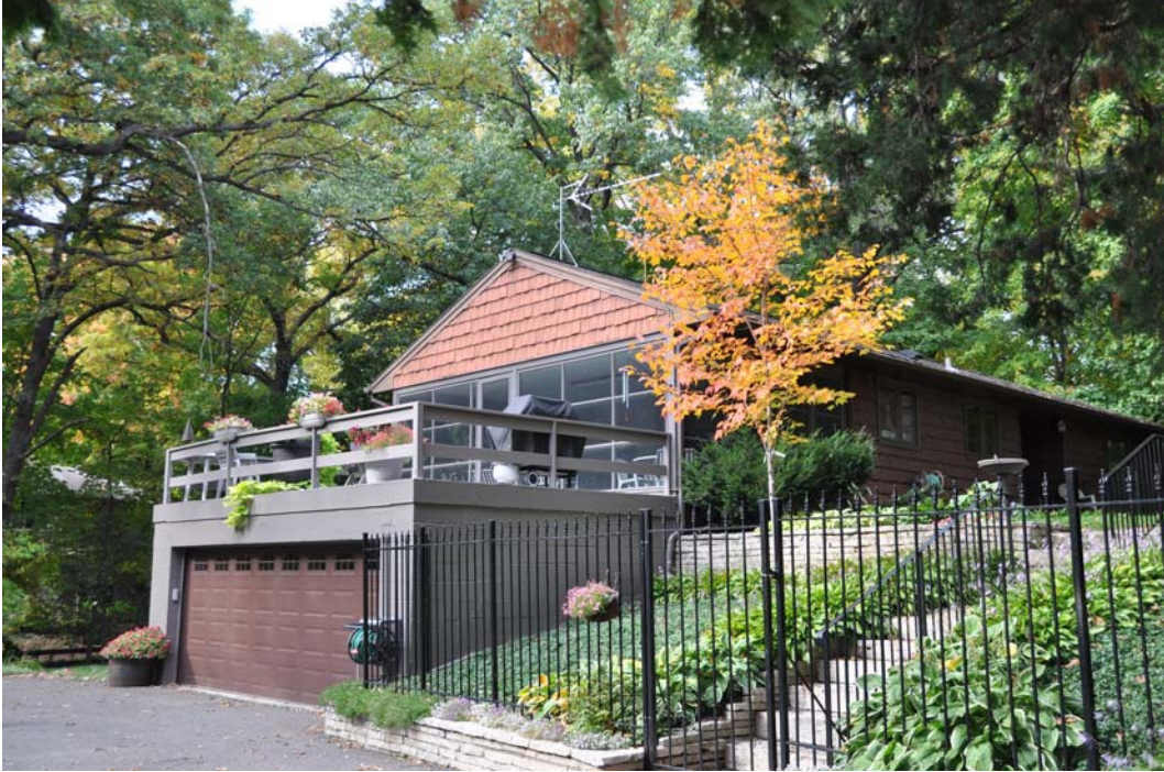
231 Bushaway Road Photograph courtesy of Ron Anderson
