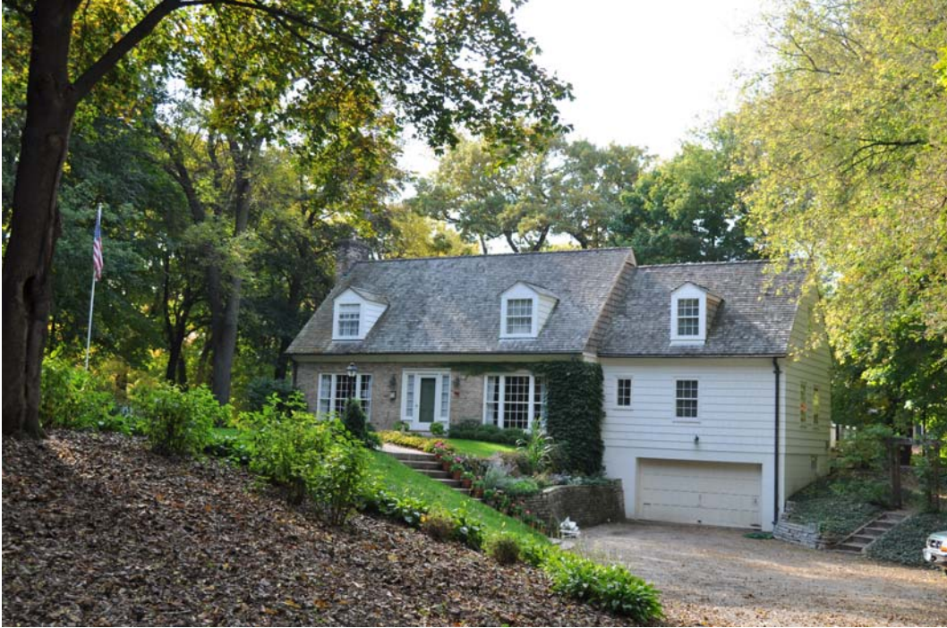
217 Bushaway Road Photograph courtesy of Ron Anderson
