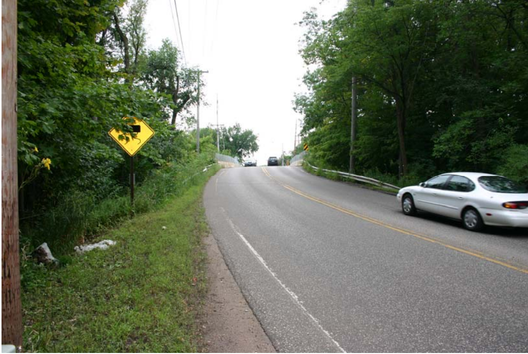
Bushaway Road – Looking south toward the bridge over the BNSF Railroad
