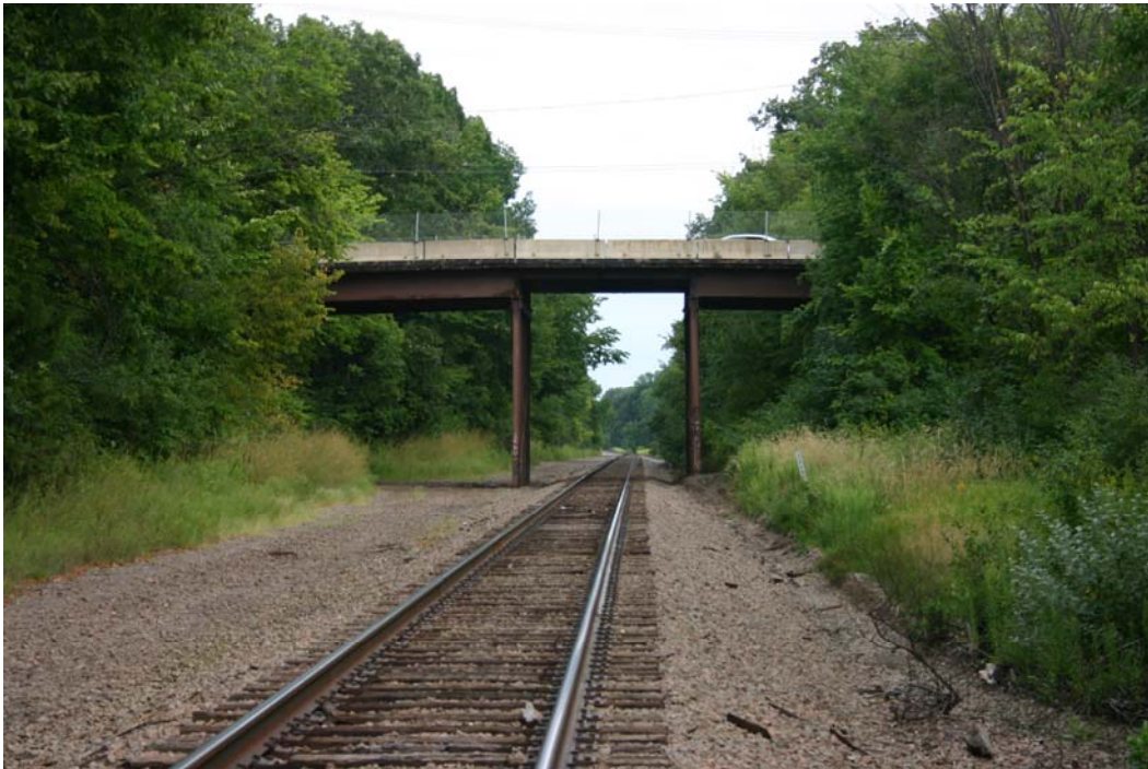
West elevation of Bushaway Road bridge over BNSF Railroad
